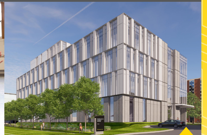
HEALTH SCIENCES ACADEMIC BUILDING: Set to be complete in summer 2025, this facility will house academic, administrative, clinical, and research space for the Departments of Communication Sciences and Disorders, Physical Therapy Rehabilitation Science, and Health and Human Physiology.
